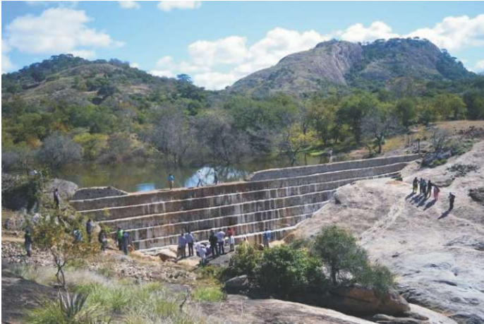
Figure 2.15: A small dam constructed by the community in Mwenezi with the assistance of the Zimbabwe Resilience Building Fund. Climate change adaptation through water harvesting and redirecting its use for agriculture, household and other uses requires hard engineering to be done.
