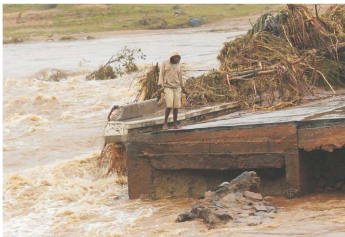
Figure 2.3 A collapsed bridge in Chimanimani pictured on 18 March 2019 in the immediate aftermath of extreme heavy rains brought about by Tropical Cyclone Idai. According to the 2019 UN Flash Appeal for Zimbabwe about 5,000 meters of the water distribution network was washed away in Chimanimani town, over 250 boreholes, 18 water supply systems were damaged and more than 50 schools lost sanitation infrastructure in Chipinge and Chimanimani districts.
