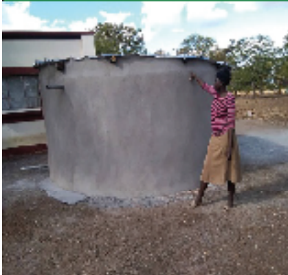
Rooftop rainwater harvesting into infiltration tank
