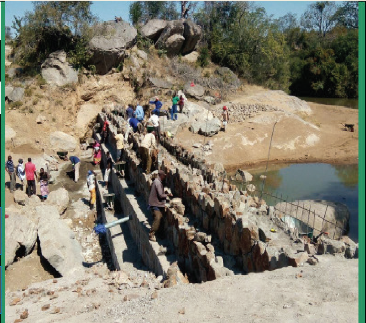
Community in Mwenezi constructing a weir for livestock and irrigation
