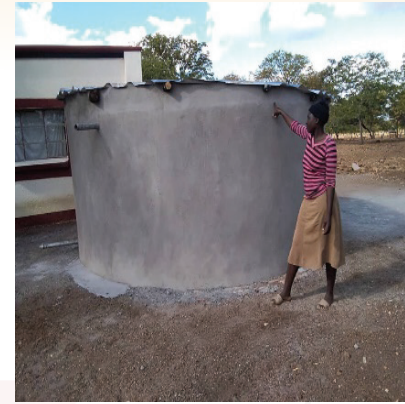
Rooftop rainwater harvesting into infiltration tank
